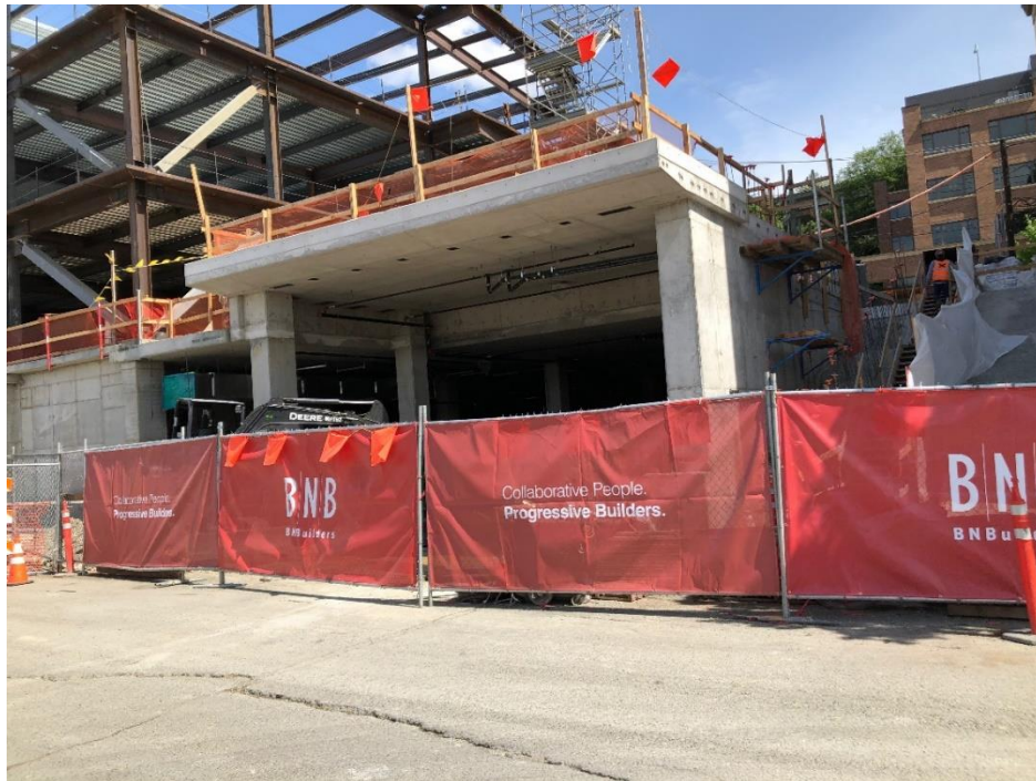
Figure 3 Photo of site fencing
