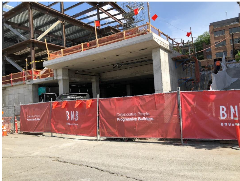
Figure 3 Photo of site fencing
