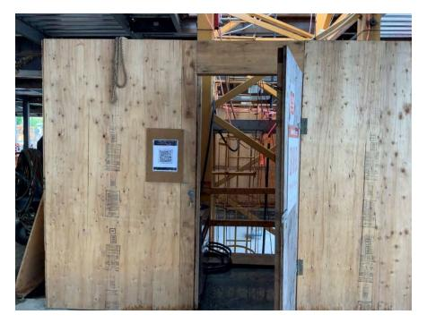
Figure 4 An access door is provided at the Tower Crane enclosure. These doors are equipped with a hasp and padlock that only the site management and Tower Crane operator are provided keys to. Doors should be locked up at the end of each day by site foreman during final walkthrough at the end of each day.
